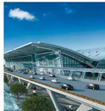
INTERNATIONAL AIRPORT SOUTH KOREA
